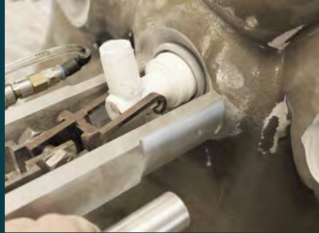
View of the jet installation system by suction
